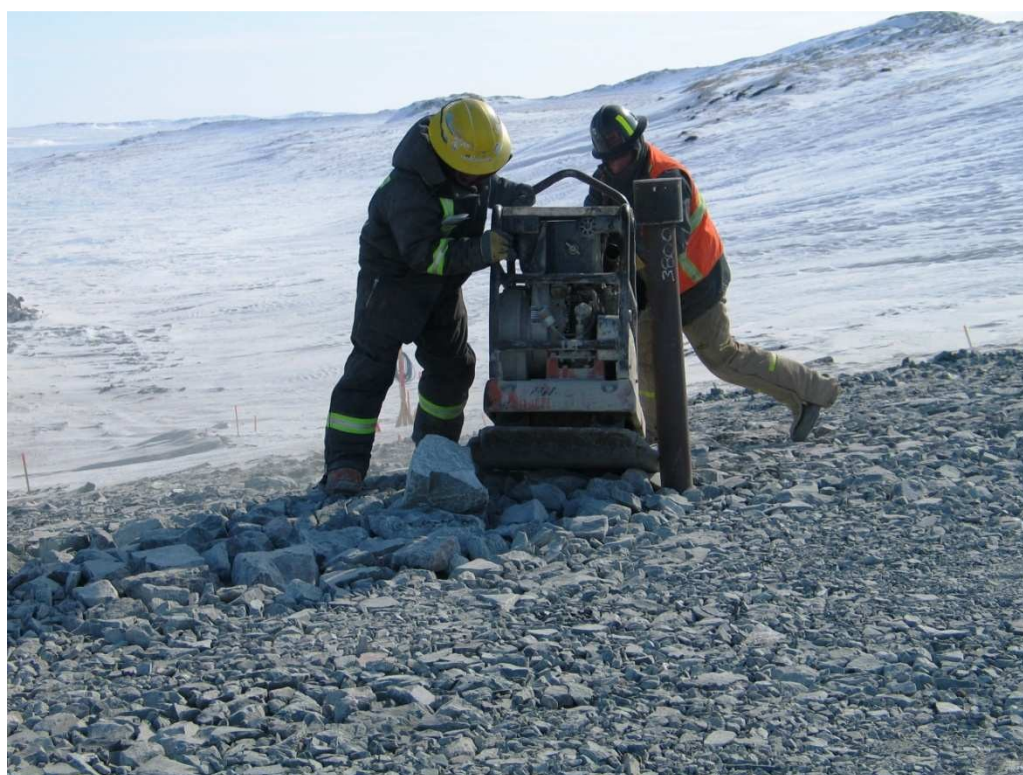
Photo 4: Packing next to the pipe was done with a hand packer
