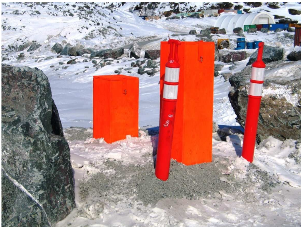
Photo 7: Junction boxes placed over thermistors at the sedimentation pond. Access through hinged lid.
