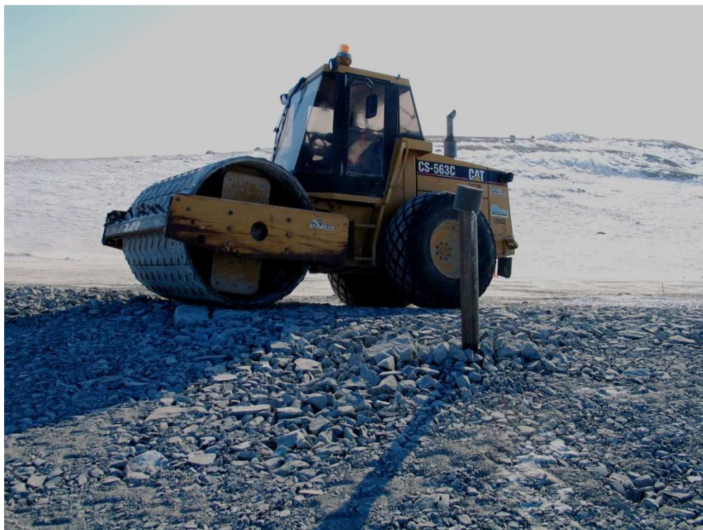
Photo 3 Final compaction was done with a 10 ton packer
