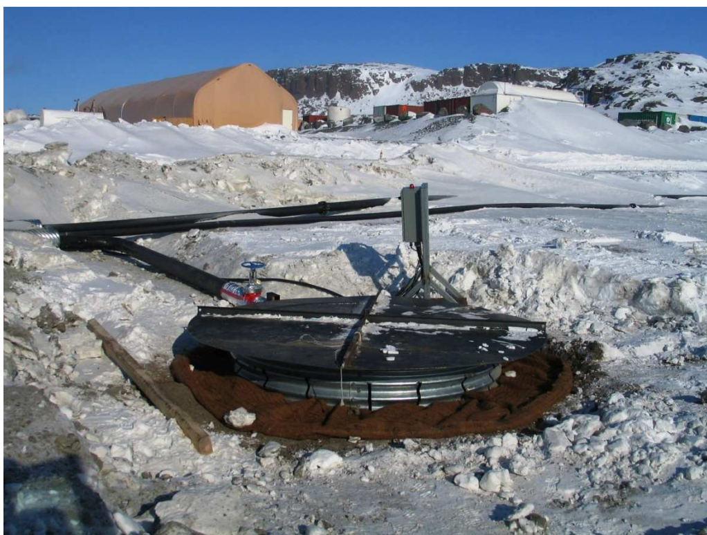
Photo 6: Coconut mats placed around Sump 2
