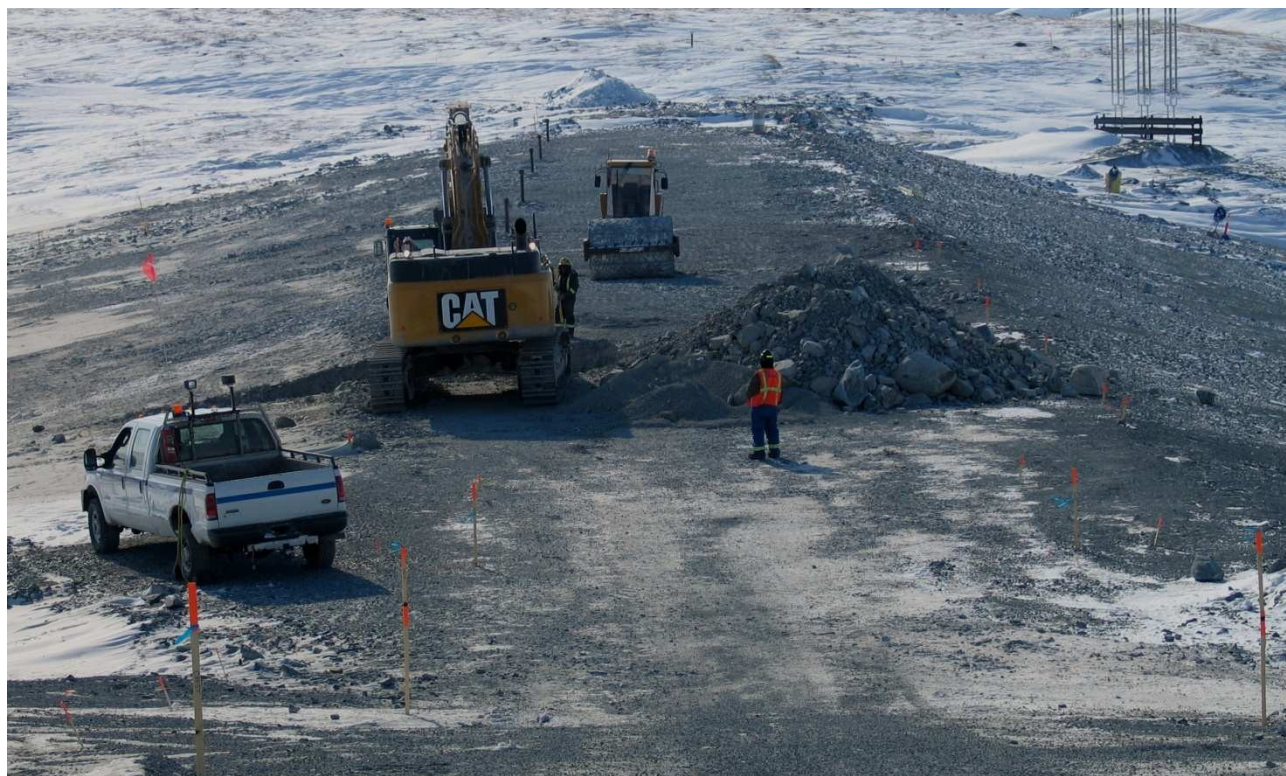
Photo 2: North dam facing south. Stakes in foreground indicate fill requirements for road onto dam
